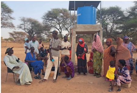
Bakary Diallo - Solaranlage & Tank
